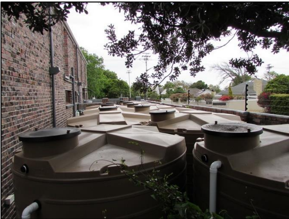
Left: The 'tank farm' – 10 x 5000 litre tanks plumbed into the house's water system. Right: A bed edged with banana tree trunks and mulched with wood shavings.
